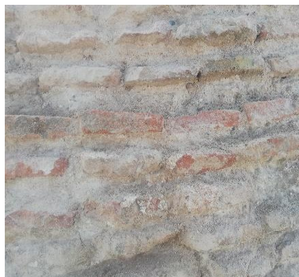
Plate 08. Gap Between Burnt-bricks Course
