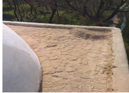
Plate 10. After Removal of Surface Material from the Floor
