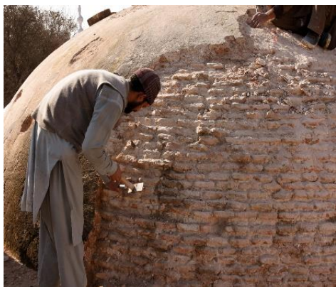
Plate 07. Removal of Loose Material from Dome
