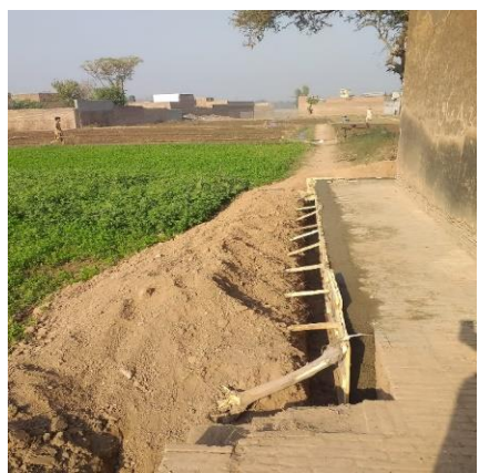
Plate 05. Platform After Concrete Filling
